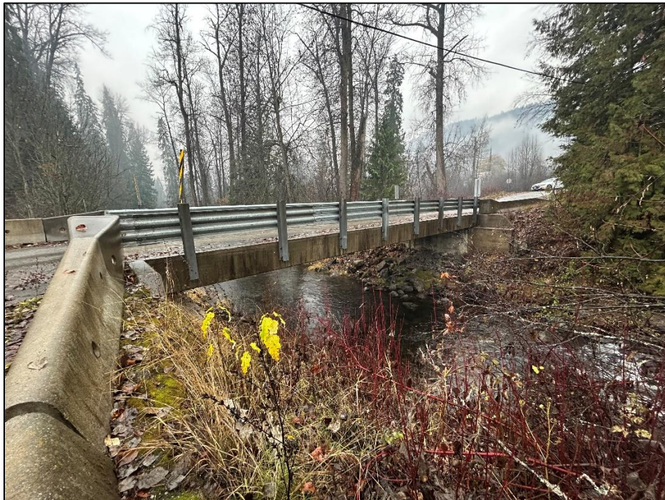
Photo C10: Jefferson Road Bridge
