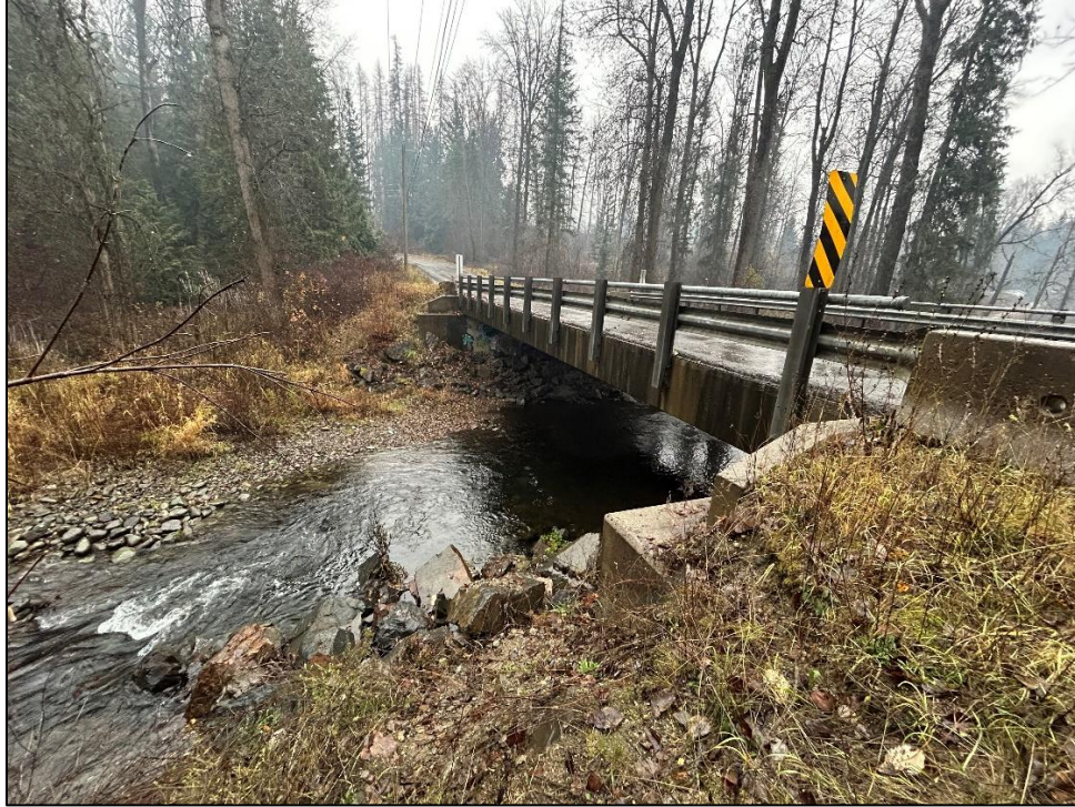
Photo C9: Bluebird Road Bridge
