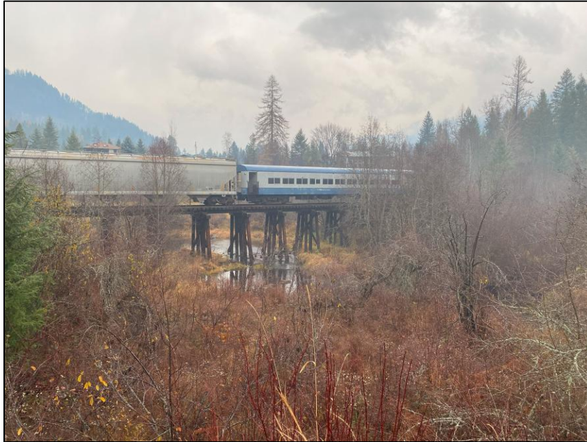
Photo C1: Railway Crossing Bridge
