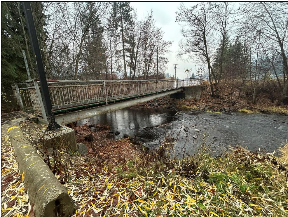
Photo C6: Beaver Street Pedestrian Bridge
