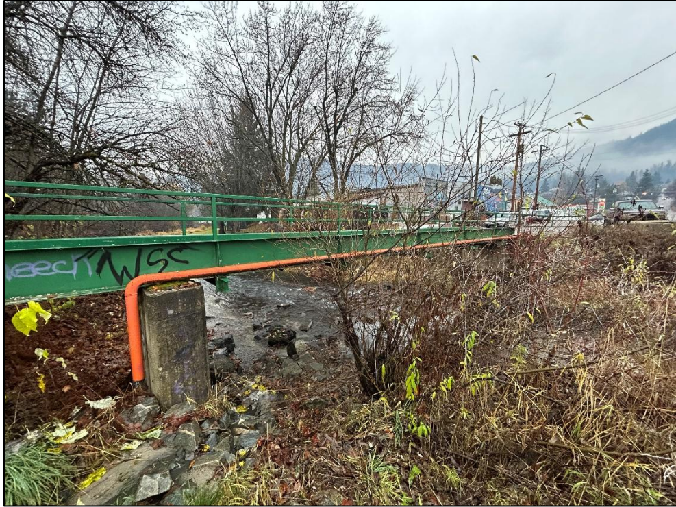
Photo C5: Kootenay Avenue Pedestrian Bridge
