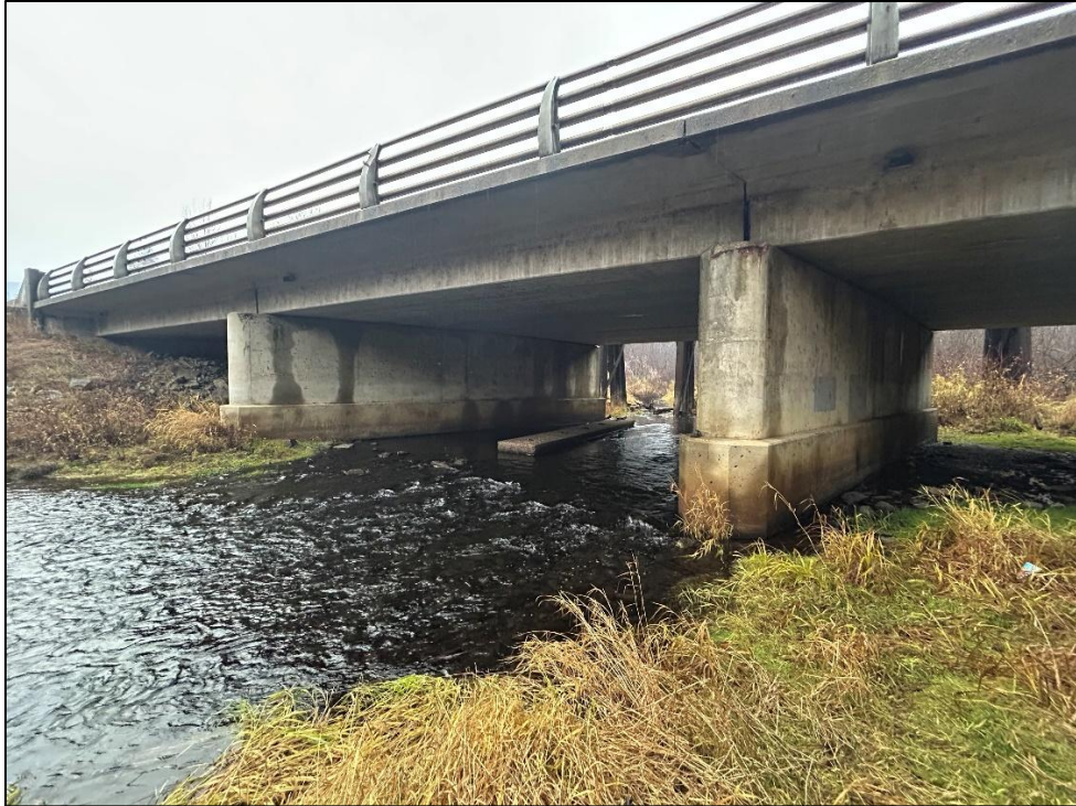
Photo C3: Current Highway 3B Bridge
