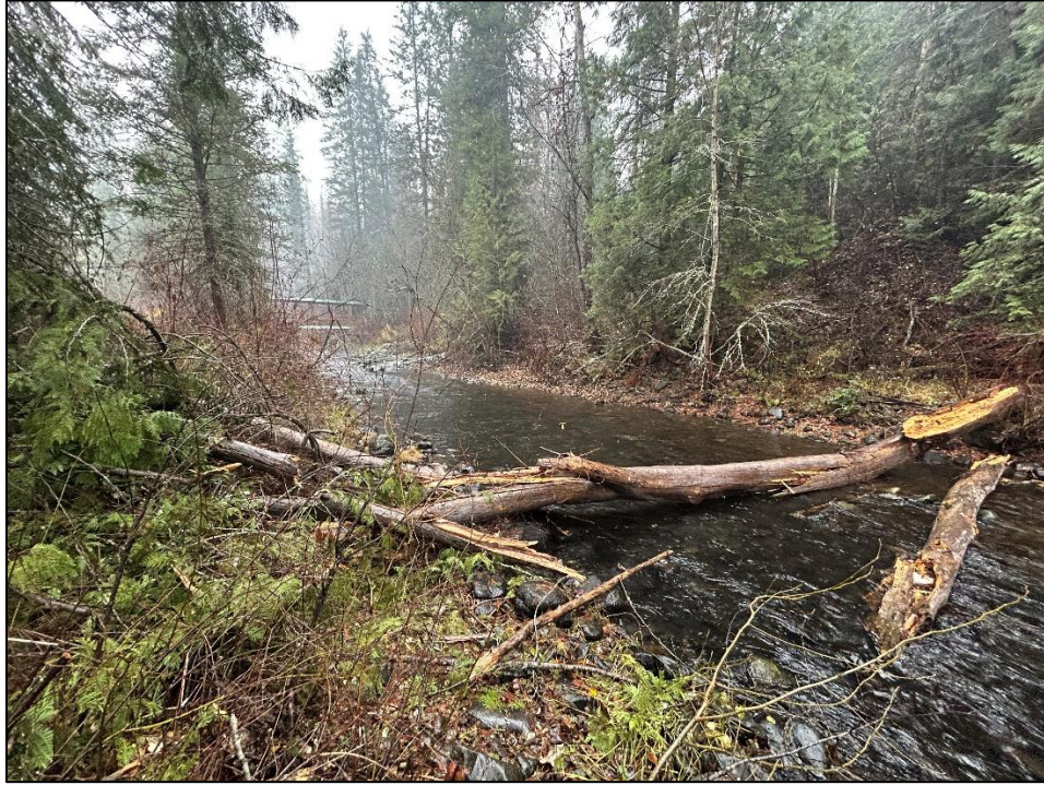
Photo C7: Camp Tweedsmuir Pedestrian Bridge (Upstream)
