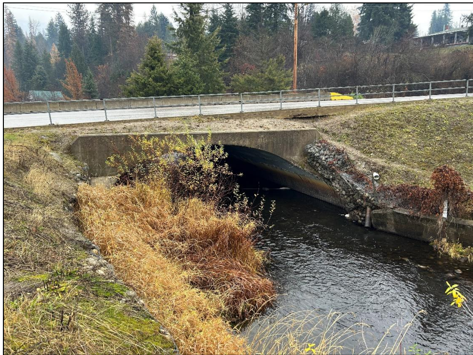
Photo C4: Columbia Gardens Arch Culvert
