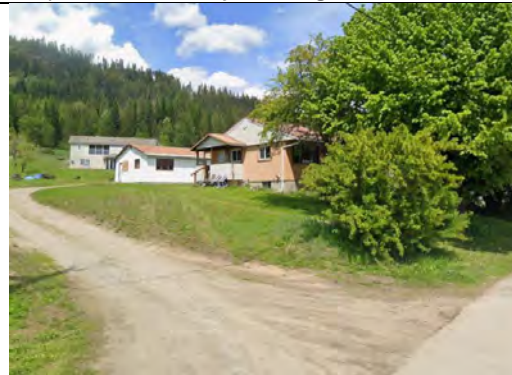
Looking east on Mountain St
