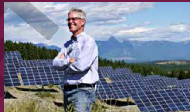
Sunmine Municipal Solar Farm, Kimberley, BC
