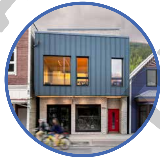
Tantrum Bike Shop in Revelstoke is a net-zero-ready building
