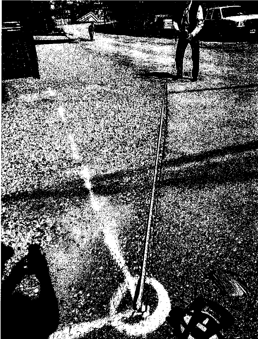
Note the ~5-m bevelled corner, with a fanned gravel boulevard widening to 2.4 m. The deck edge and spray-painted line marks the property boundary. Stormwater from Kootenay Ave South percolates into the permeable boulevard surface. The side yard slopes upward from the street toward the building.
