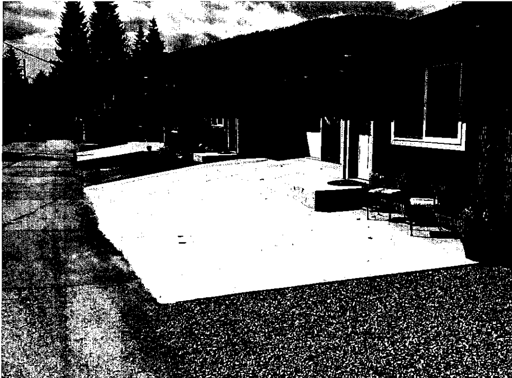
Looking west on Kootenay Lane. All north side (lower side) properties' front boundaries abut the road asphalt and witness stormwater flow. The property at 1897 has a frontage area that slopes upward to the building, neutralizing stormwater flow impacts.
