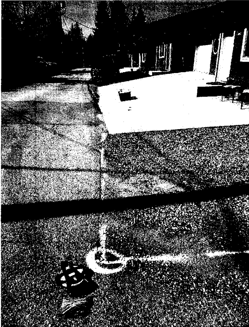
Demarcated 4.2-m property boundary along Kootenay Lane and upward slope toward the residence at 1897 Kootenay Lane. The property pin is circled. The grade where Kootenay Lane intersects with Kootenay Ave South conveys the stormwater toward Kootenay Ave South. The existing road grit shows the flow patterns clearly.
