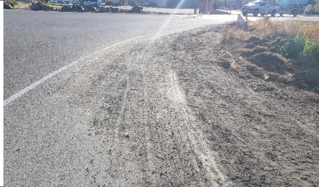
NORTHWEST side looking SOUTH – Note painted white disappears. This is misleading as it appears as though there is no paved shoulder
