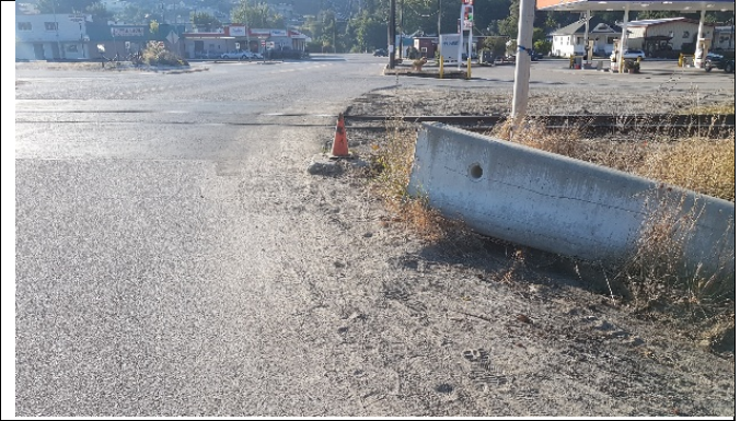
NORTHWEST side looking SOUTH – Note painted Orange safety cone. There is concrete foundation square which the No-Post probably used to protect vehicles from hitting? White line non-existent. Should be 3-5 feet from the edge of the paved shoulder and carry onto Main Street.
