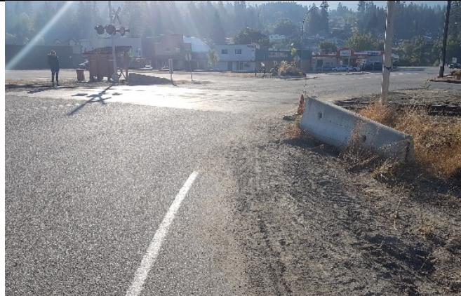
NORTHWEST side looking SOUTH – Note painted white disappears. This is misleading as it appears as though there is no paved shoulder. No-Post is completely off the road and halfway into ditch
