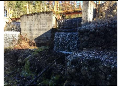
Photo #15: Gabion basket on south abutment show signs of settlement and movement away from concrete wall, but appear to be consistent with previous years.
