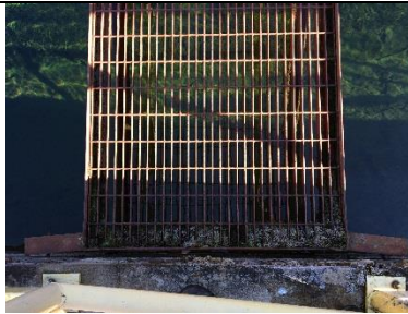
Photo #17: Steel platform connection members exhibit shear failure and connection failure.
