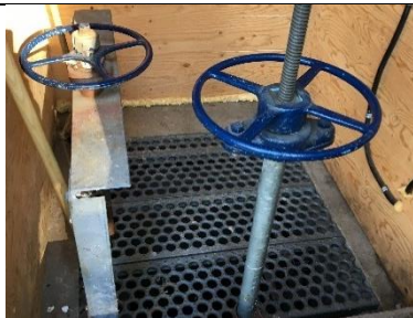
Photo #20: Intake valves and housing.
