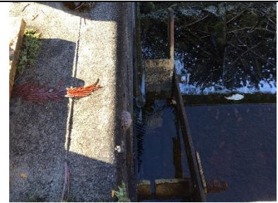
Photo #18: Rubber side seal damaged on south side of southern spillway gate.
